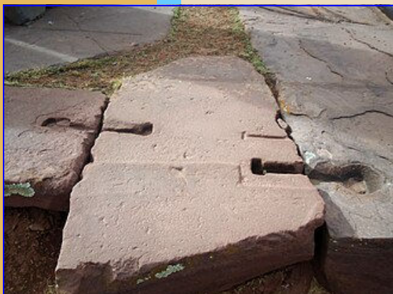
Fig. 7. Joint groups floor foundation, monolithic blocks, fastened together with special clamps at Puma Punku 5,240 miles from Montana. Wikimedia Commons.
