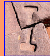
Double-T style stone clamp cuts, ancient Bolivia
