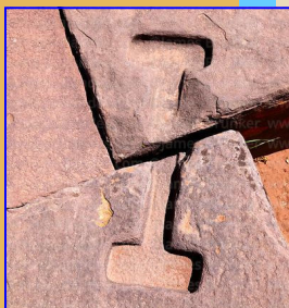
Fig. 8. Clear "double-T" or "dumbbell"-style clamp cut, Puma Punku, per the styles discussed in the comprehensive 2020 paper by Kim Hongnam. Magical Andes Photography.
