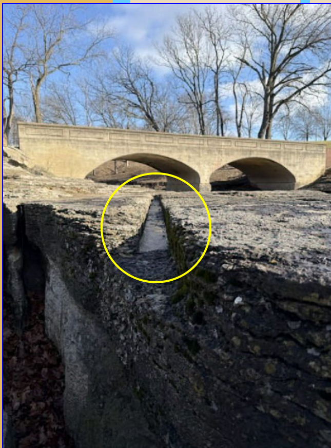
Fig. 3. View of slabs and groove in the creek bed. Some have mused that perhaps the straightness and flatness of everything was a result of the mill installation at the Falls in the 1850's, without proposing what their purposes might have been. This is not a credible argument because a recent cutting of the rock slab and the ruts show the same patina as the flat slab surface. Photo: Carl Adam Carter; circle added.
